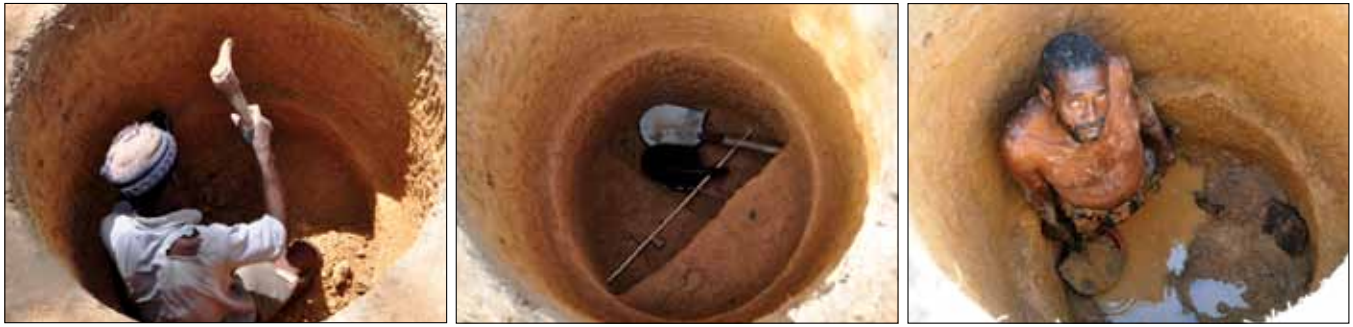
GARDEN WELLS: These photos show the progress of a hand-dug well, along with the tools used in the project.
